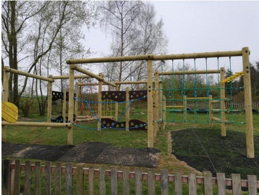
The new KS1 frame
